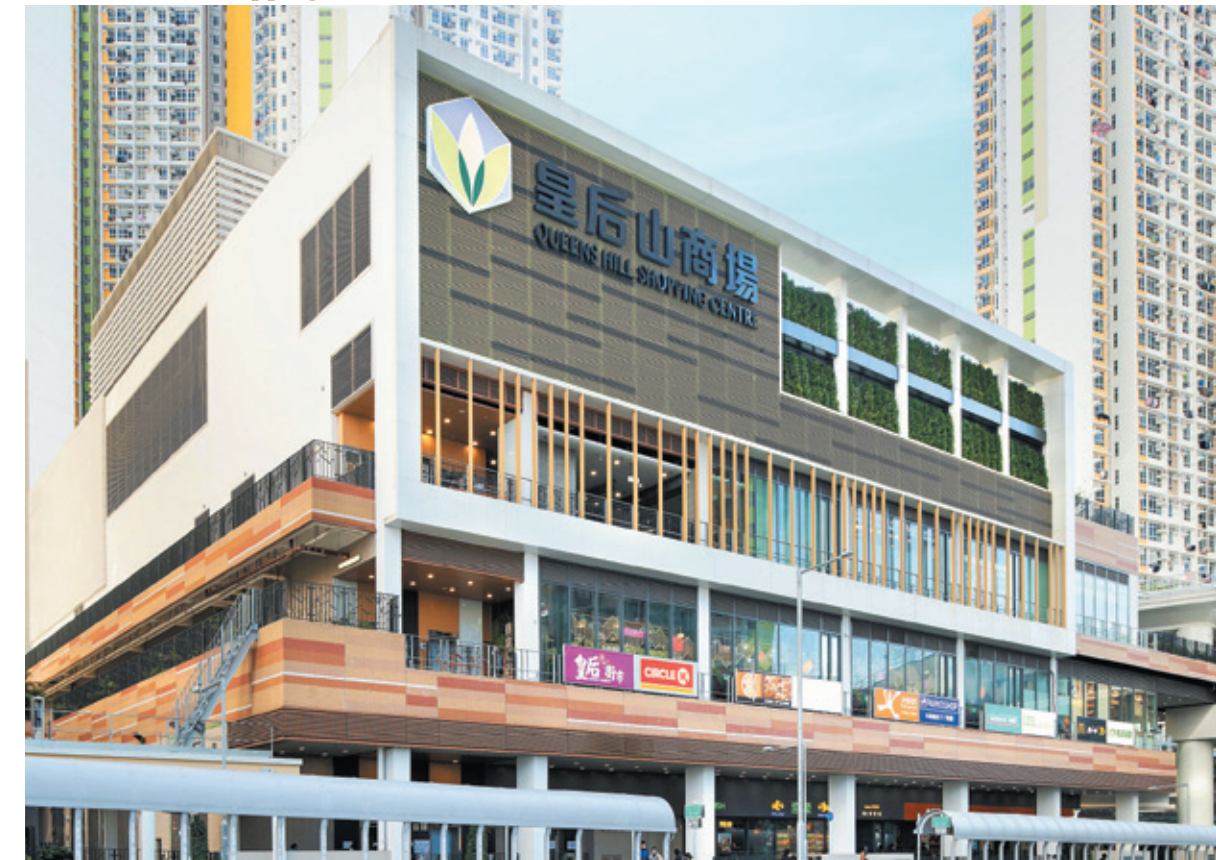
▼ Queens Hill Shopping Centre
