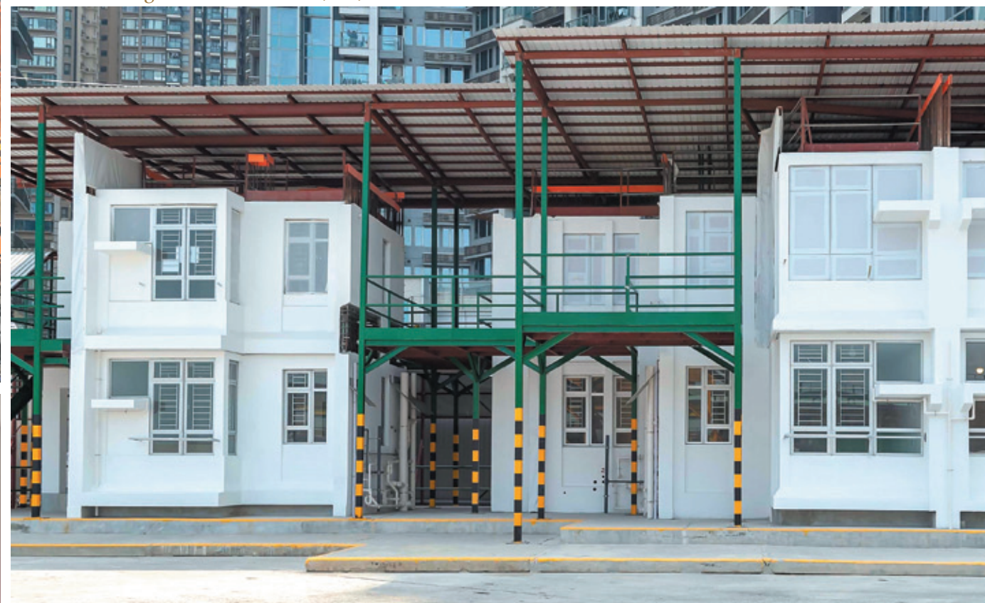
▼ Modular Integrated Construction (MiC)
