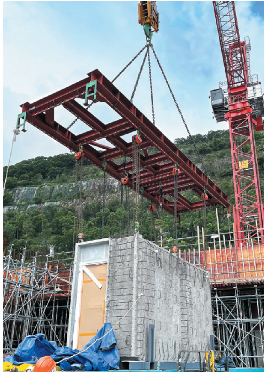
▲ Modular Integrated Construction (MiC)
