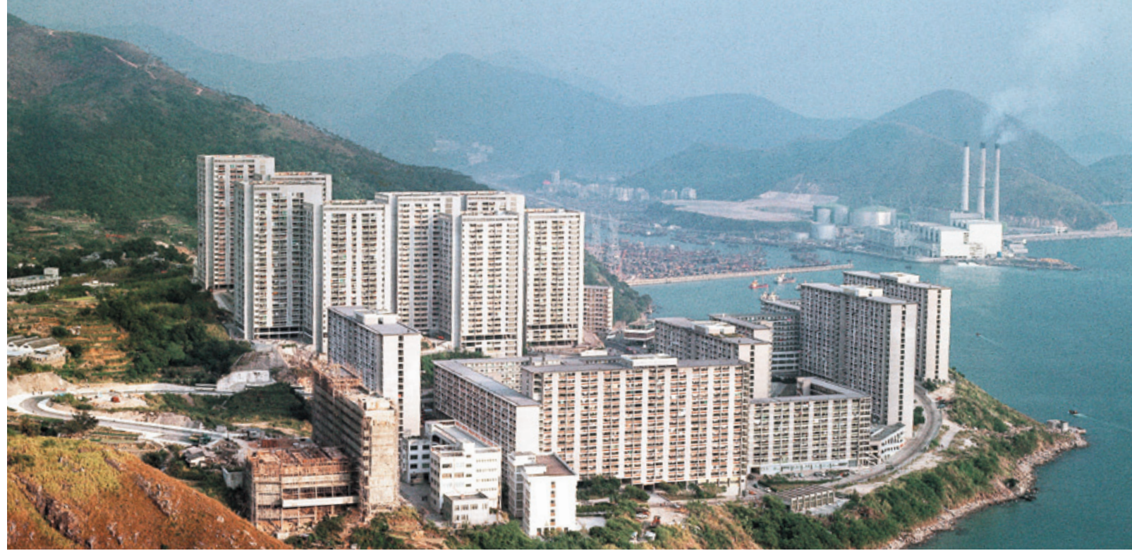
▲ Twin Tower blocks (Wah Fu Estate)
