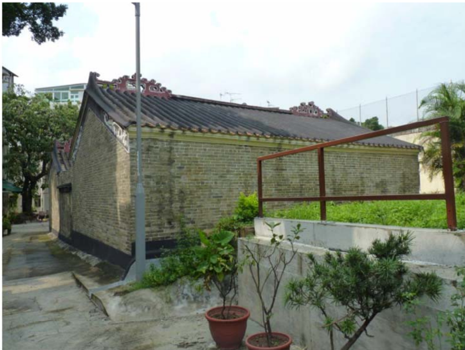
Rear Elevation of the I Shing Temple
