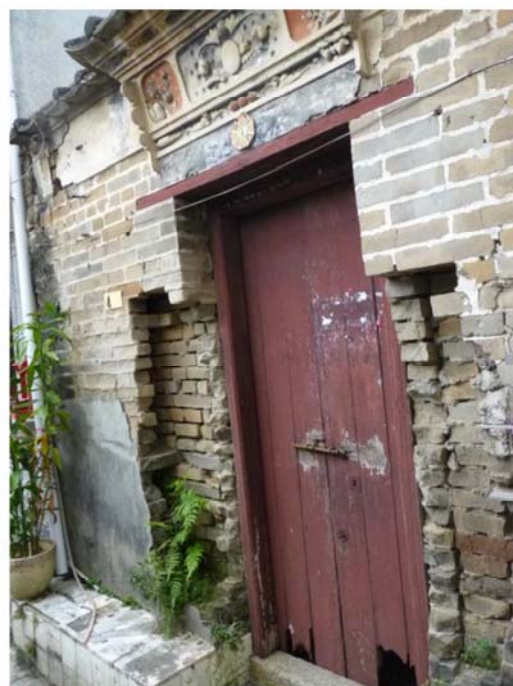
Detail View of the Façade of No. 4
