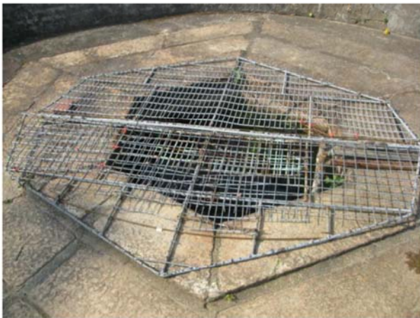
Detail view of the well opening
