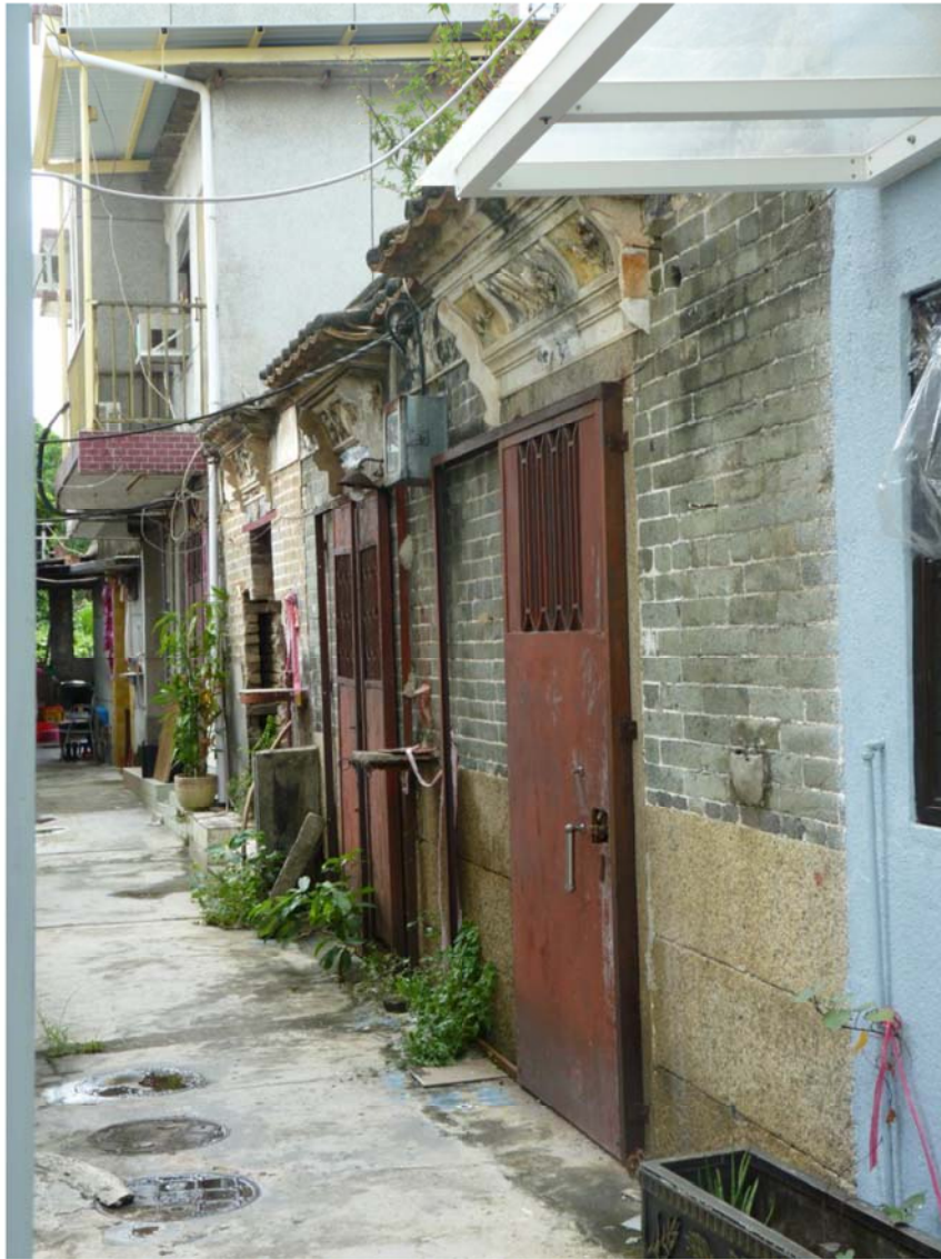
View of the façade of the buildings (No. 7A in the foreground)
