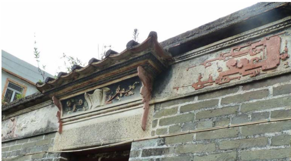
Detail View of Door hood and decorative Frieze panel of no. 41 Shing Uk Tsuen
