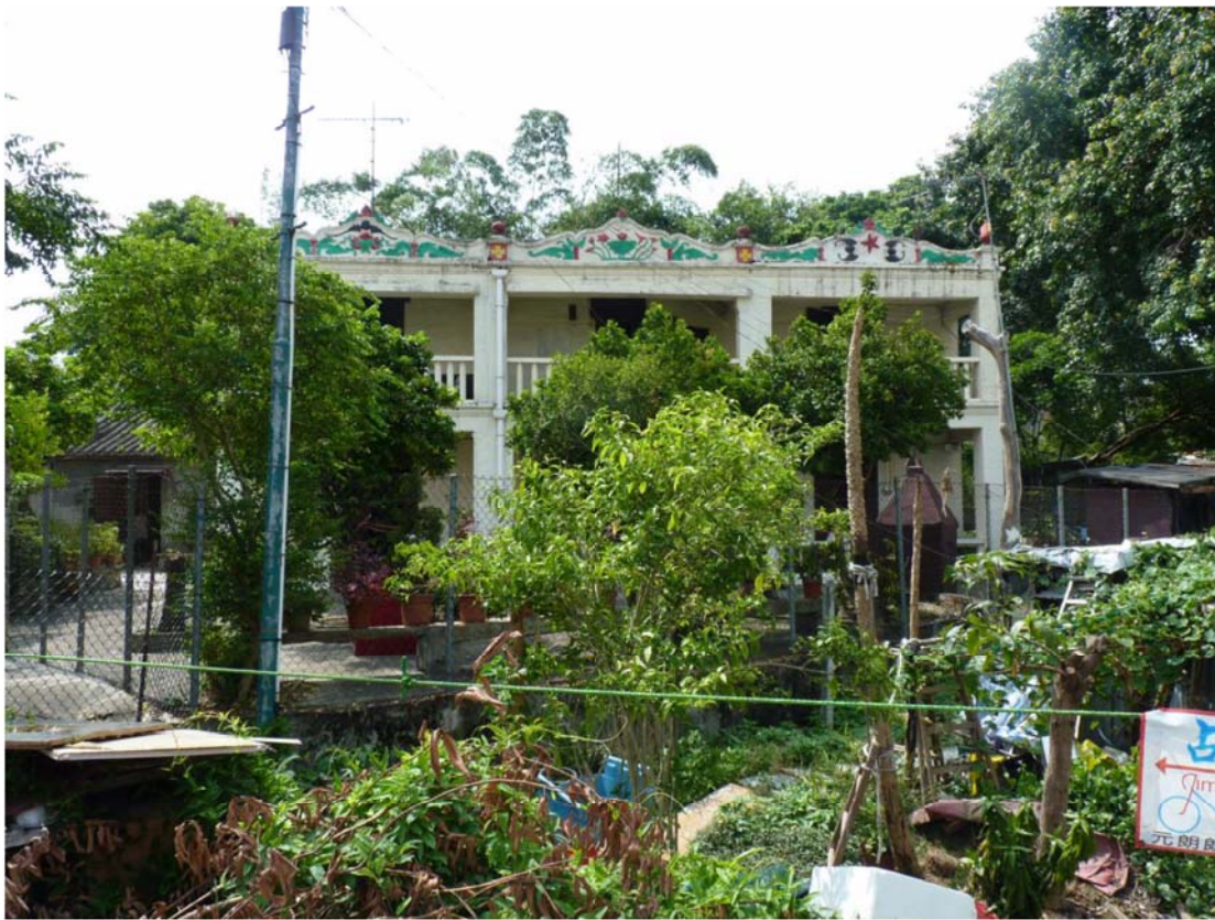
General View of the building
