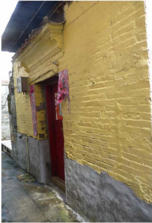
Façade of No. 41 Fuk Hing Tsuen
