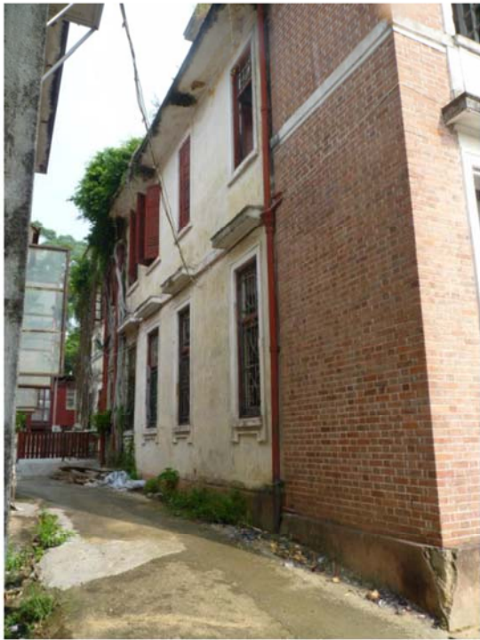
View of the Southwest Elevation of Yu Yuen Mansion
