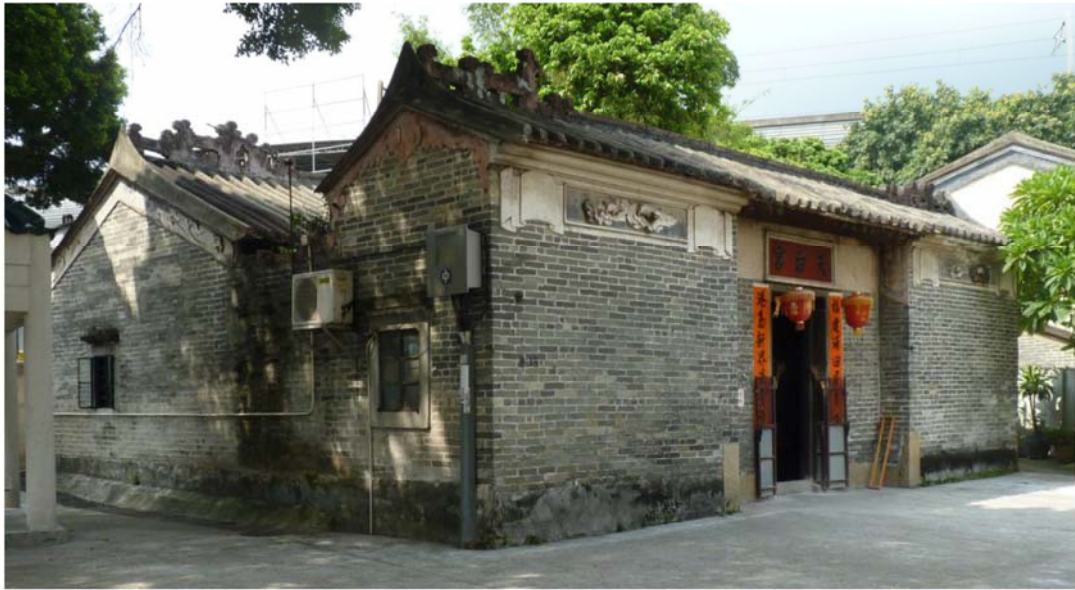
Façade and Southwest Elevation of the Tin Hau Temple in Fung Chi Tsuen
