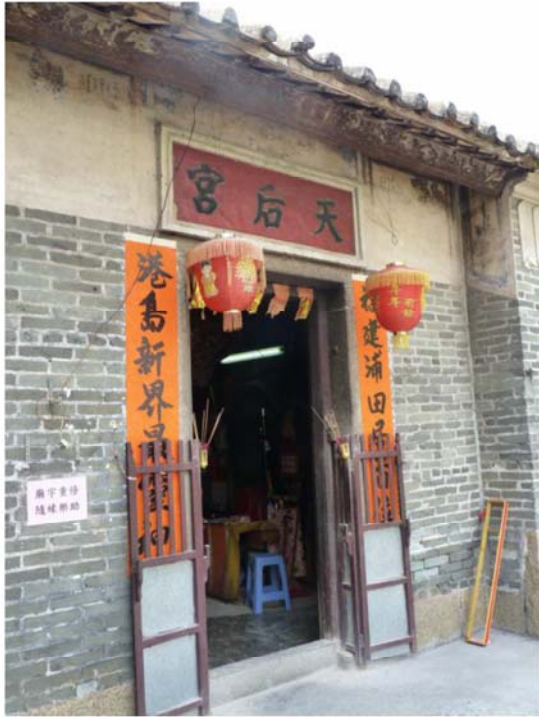
Detail View of the Entrance to the Tin Hau Temple in Fung Chi Tsuen
