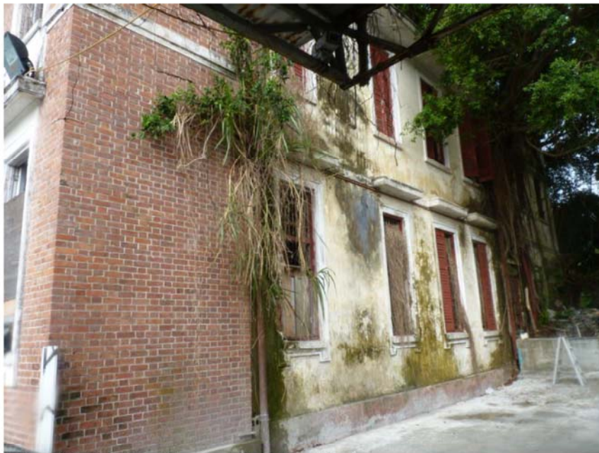
View of the Northeast Elevation of Yu Yuen Mansion
