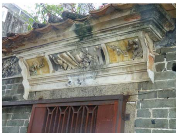
Detail View of the Door Hood of 7A
