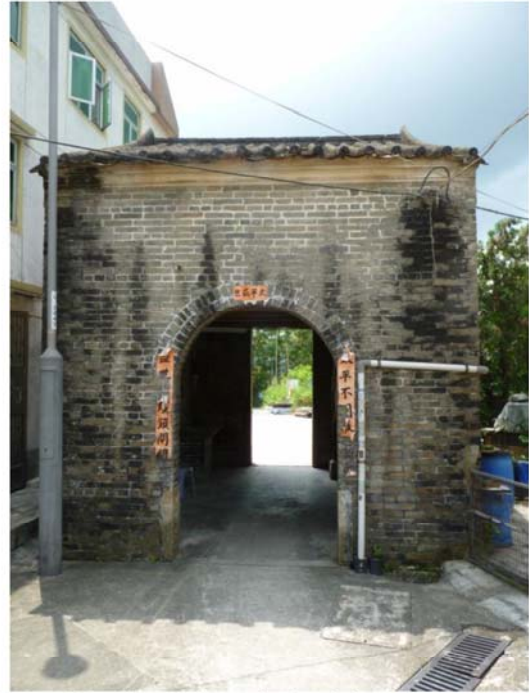
Rear (Northern Elevation) of the Entrance Gate
