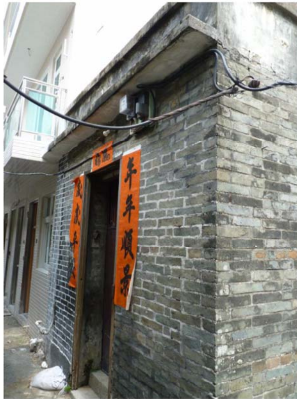
Façade of No. 40 Fuk Hing Tsuen
