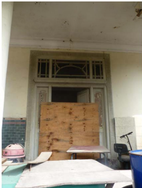
The Main Entrance of Yu Yuen
