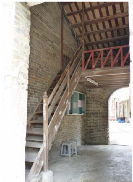
Staircase and Cockloft in the Entrance Gate
