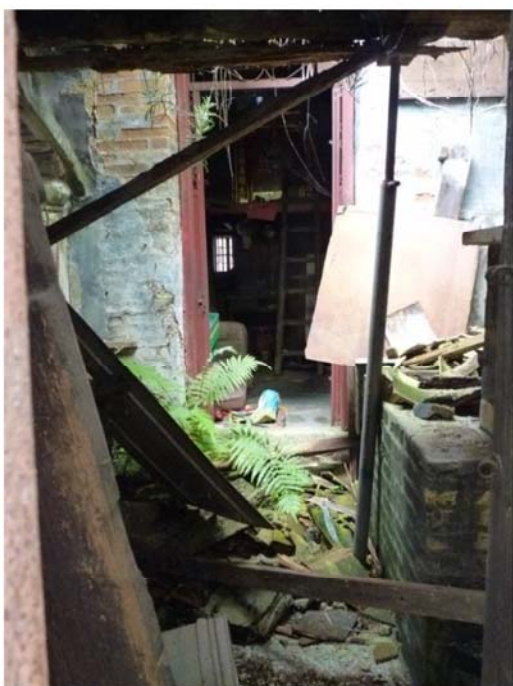
Detail View of the Interior of Lot WCL132 in DD123
