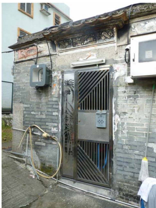
Façade of No. 39 Shing Uk Tsuen
