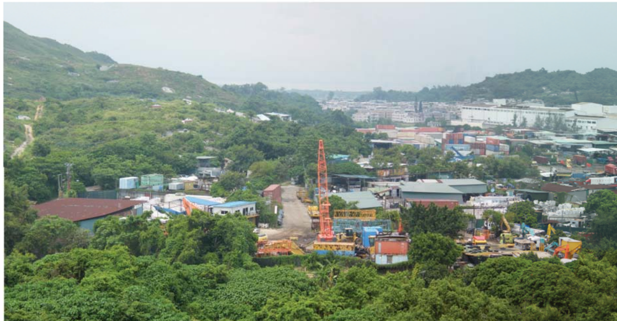
VSR 16: Foothills above Yeung Uk San Tsuen
