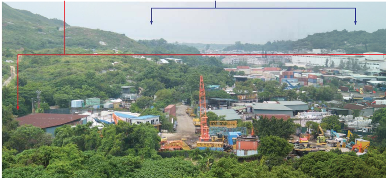
VSR 16: Foothills above Yeung Uk San Tsuen
